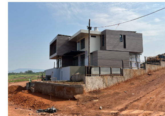
Above: Side view of the Single Residence (January 2023)
